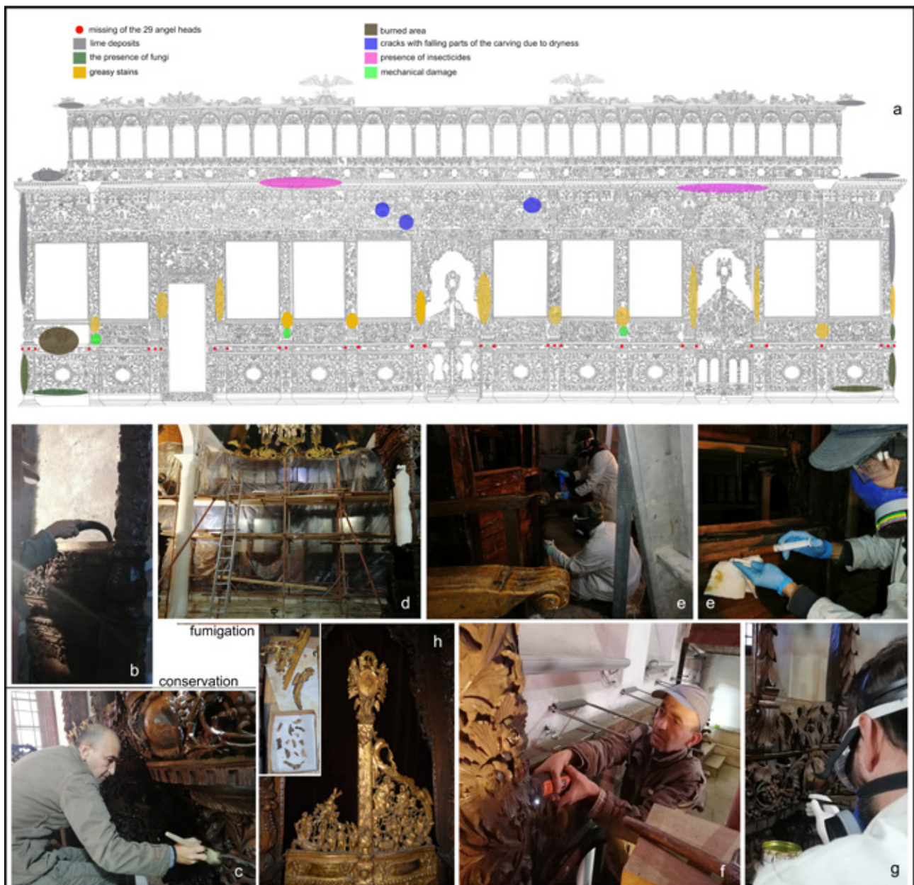
Fig. 2 - The type of damages and the processes of conservation on the iconostasis:
